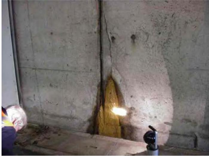
Figure 3 Cracking at segment joint
